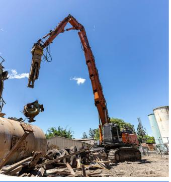
Precision engineering was required for demolition of the uncontaminated crystallisation tanks, which weighed approximately 700 tonnes. The tanks were demolished using the induced collapse method, a process which was facilitated by oxy cutting the flooring to create sufficient room for the tanks to fall. Once on the ground, the tanks were pulled from the shed using the 30 and 35 tonne excavators.
