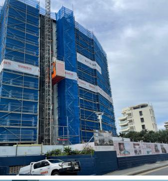
The original methodology was designed as a top down demolition to level three followed by use of the 52 tonne high reach excavator for deconstruction of the remaining levels. This methodology was revised due to the limited space on the 1.600m2 site.
