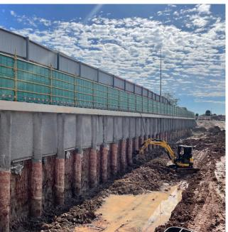
Ascot Green by Mirvac is located in Brisbane's northside. As part of ongoing residential developments, DEMEX was engaged by Mirvac to undertake bulk earthworks, shotcreting, installation of FRP capping beams, stormwater works, and other minor site works for Tower C (Charlton House) of the development; the third tower in the series.
