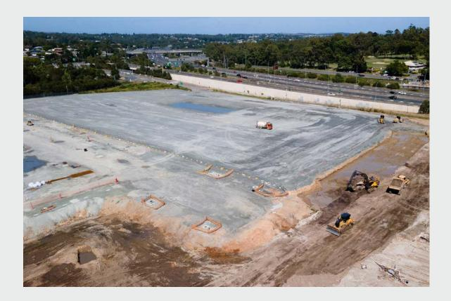
The client requested early contractor involvement on the demolition associated civil work for this project. In consultation with a specialist geotechnical engineer, DEMEX undertook a baseline test across the site to establish the conditions of materials. It was evident that a graduated build up was needed to meet the site construction requirements and that suitable material must be sourced to construct a wearing course to bulk earthworks level for handover to the builder.
