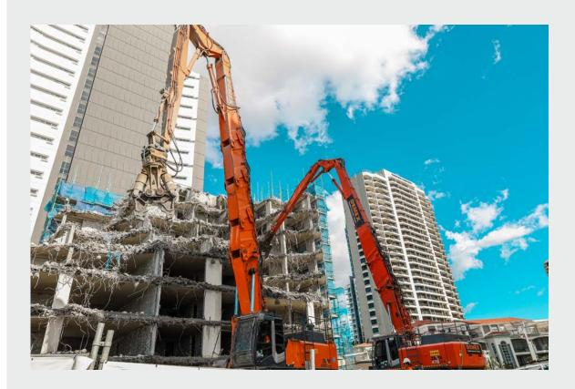
DEMEX commenced this project – demolition of an eight storey highrise using a top down method - approximately one month prior to signing a contract under an ECI agreement. At this point, ECI was implemented solely around methodology for demolition works.
