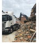
BALLINA HIGH SCHOOL Engaged as the principal contractor, DEMEX completed the demolition and extensive hazmat at a large school block on the Ballina High School campus. The project included the removal of blackjack vinyl adhesives, window mastics and PCBs'.
