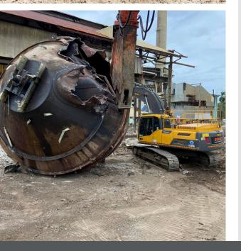
DEMEX was engaged to undertake demolition of the crushing house, tank farms, factory workshops and offices, molasses tank, clarification tanks, processing area, sugar storage shed, and tanks. Asbestos removal works also formed part of the project scope.
